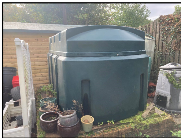
Exterior fuel storage tank
